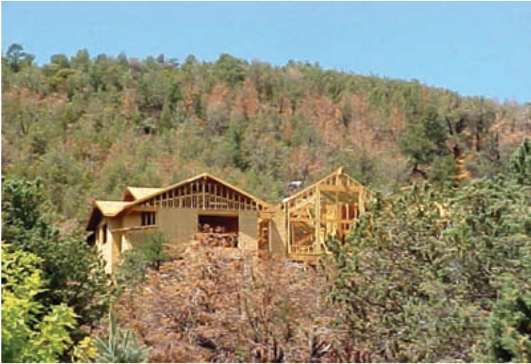
Figure 19. New home construction in a potentially hazardous setting near the Tonto National Forest.
