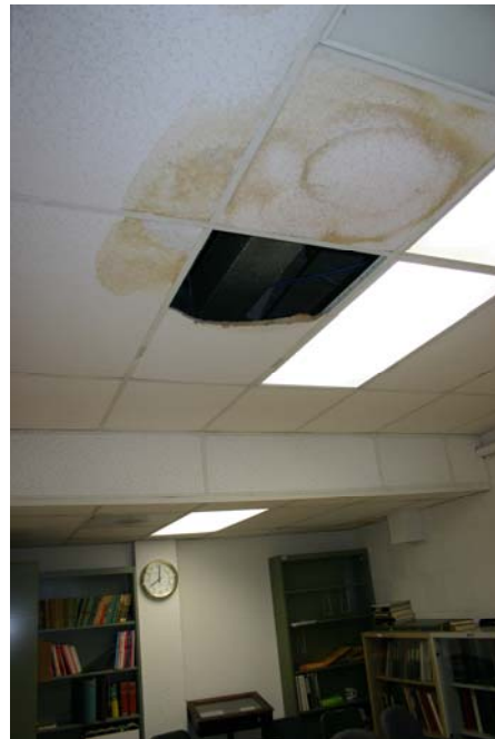
Chronic leaking through the concrete bleachers overhead repeatedly ruins ceiling tiles and damages research and teaching materials in our offices and labs.
