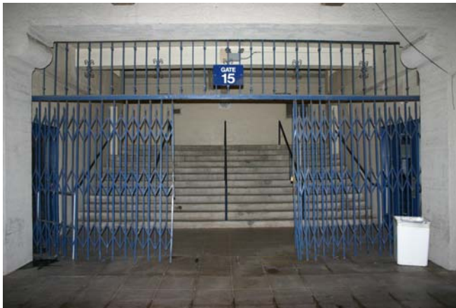
Entrances to steps and the 2 nd floor have rickety, old metal gateways that are closed and locked between 5PM and 8AM, making entry/exit difficult for staff and faculty after hours, and a hazard in case of emergencies.
