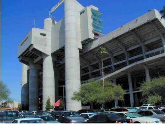
West Stadium. The “sky boxes” were added in the 1980s.
