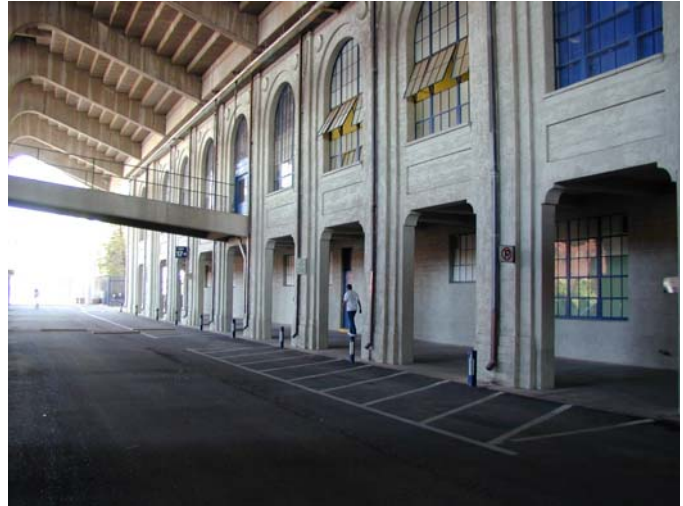
The Tree-Ring Lab occupies most of the 1 st and 2 nd floor of the old building, which was built in 1929.
