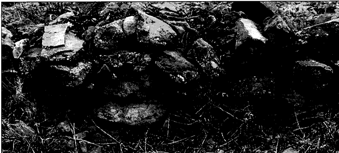
Figure 5.37: Typical Cerro Colorado wall
