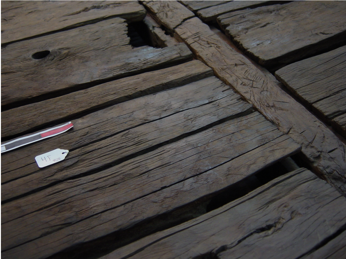
Figure 50. Tool marks on throughbeam 3 and deck planks in section 4 (room D) of GC 4926 (P. Creasman).
