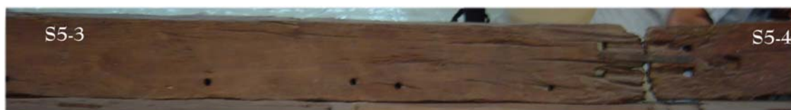
Figure 42. Inboard surface of S5-3 and its joint with S5-4 (P. Creasman).
