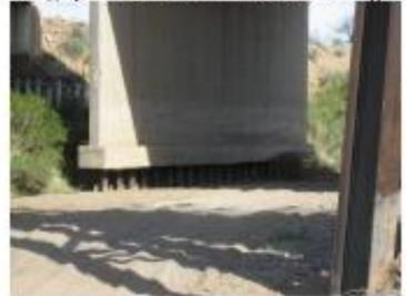
Scour of Pima Mine Road Bridge piers. The Scoured bank upstream of Pima Mine Road bottom of the pier base (top of pile shafts) is now 3 feet above the channel but was originally 6 feet below the channel bed when built in 1969-1970.
