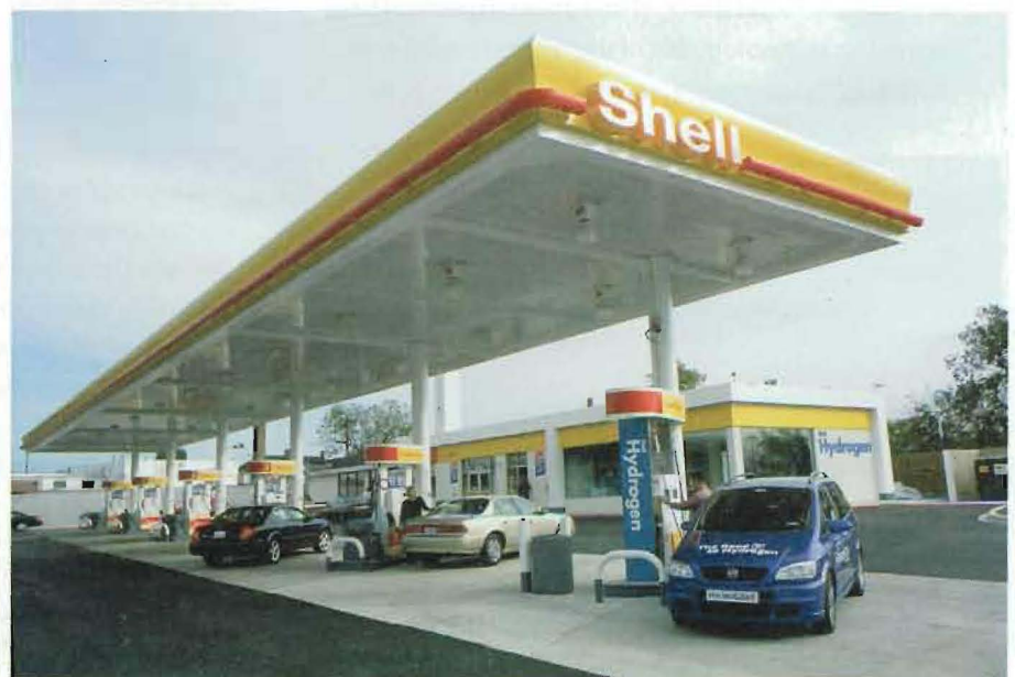
Shell Hydrogen and General Motors teamed up to build the first combined hydrogen and gasoline fueling station in North America, located in Washington, DC.
