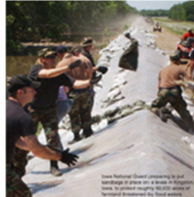
Iowa National Guard preparing to put sandbags in place on a levee in Kingston, Iowa, to protect roughly 50,000 acres of farmland threatened by flood waters.
