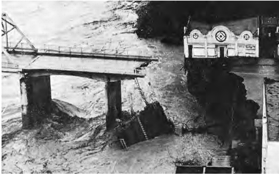
Figure 28. Destroyed highway bridge over Eel River at Scotia, California, following 1964 flood.
