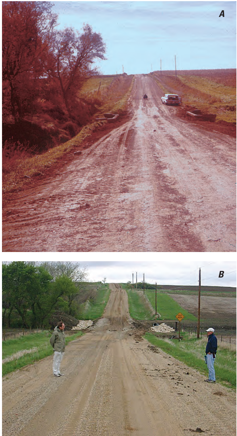
Figure 31. (A) view looking toward left bank at road and culvert crossing at Stratton Creek near Washta, Iowa, August 1961. Person on opposite bank is holding survey rod at high-water mark. (B) view looking toward left bank at road and culvert crossing at Stratton Creek near Washta, Iowa, May 2003. People standing at approximate high-water mark on right bank. Flow was from left to right.
