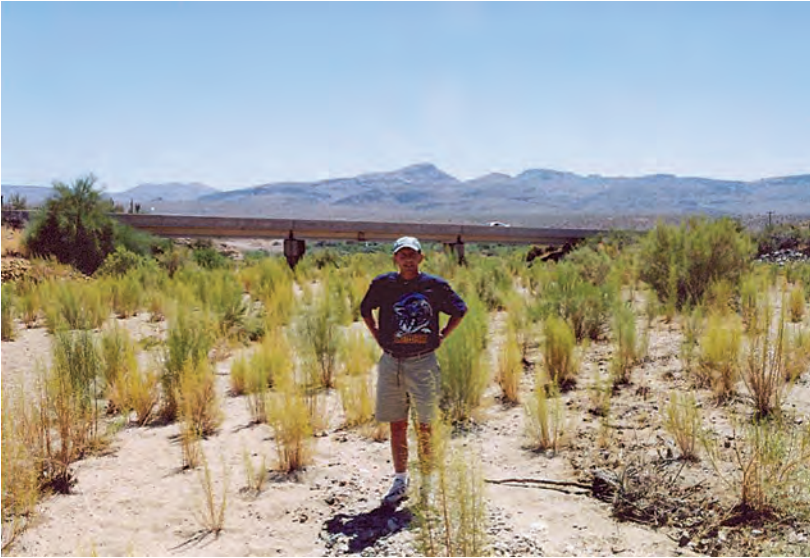
Figure 13. View looking downstream of slope-area reach toward State Highway 93 bridge across Bronco Creek near Wikieup, Arizona.
