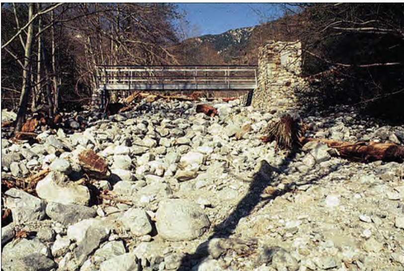
Figure 4. Deposits filling weir at Day Creek near Etiwanda streamflow-gaging station, California, February 7, 1969. View is looking upstream.
