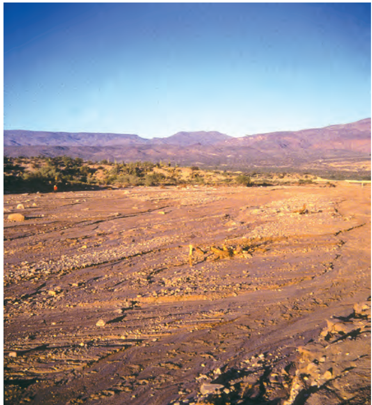
Figure 12. View looking downstream following flood in 1971, Bronco Creek near Wikieup, Arizona. Note highway bridge in upper right background where waves overtopped the road.
