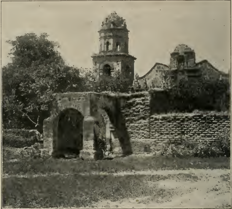
Church at Santa Cruz de las Flores, One of the Oldest Buildings in Jalisco.
