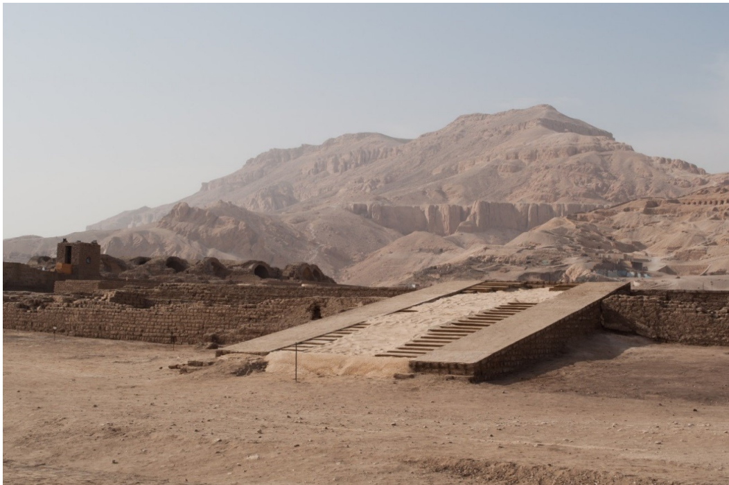
Figure 4: The ramp leading to the columned courtyard after consolidation work (photograph © T. Quirino, CEFB)
