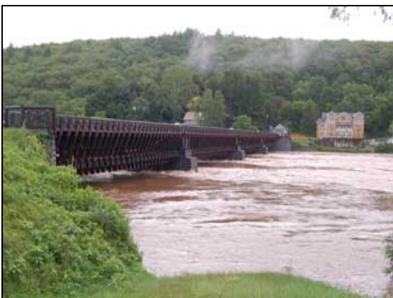
Figure 5. June 2006 flood in Lackawaxen, PA at the Roebling Bridge. (“Photo Gallery”, 2006)
