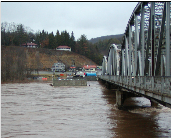
Figure 3. April 2005 flood in Barryville, NY (Courtesy of Shohola Bridge Project, Shohola, PA)
